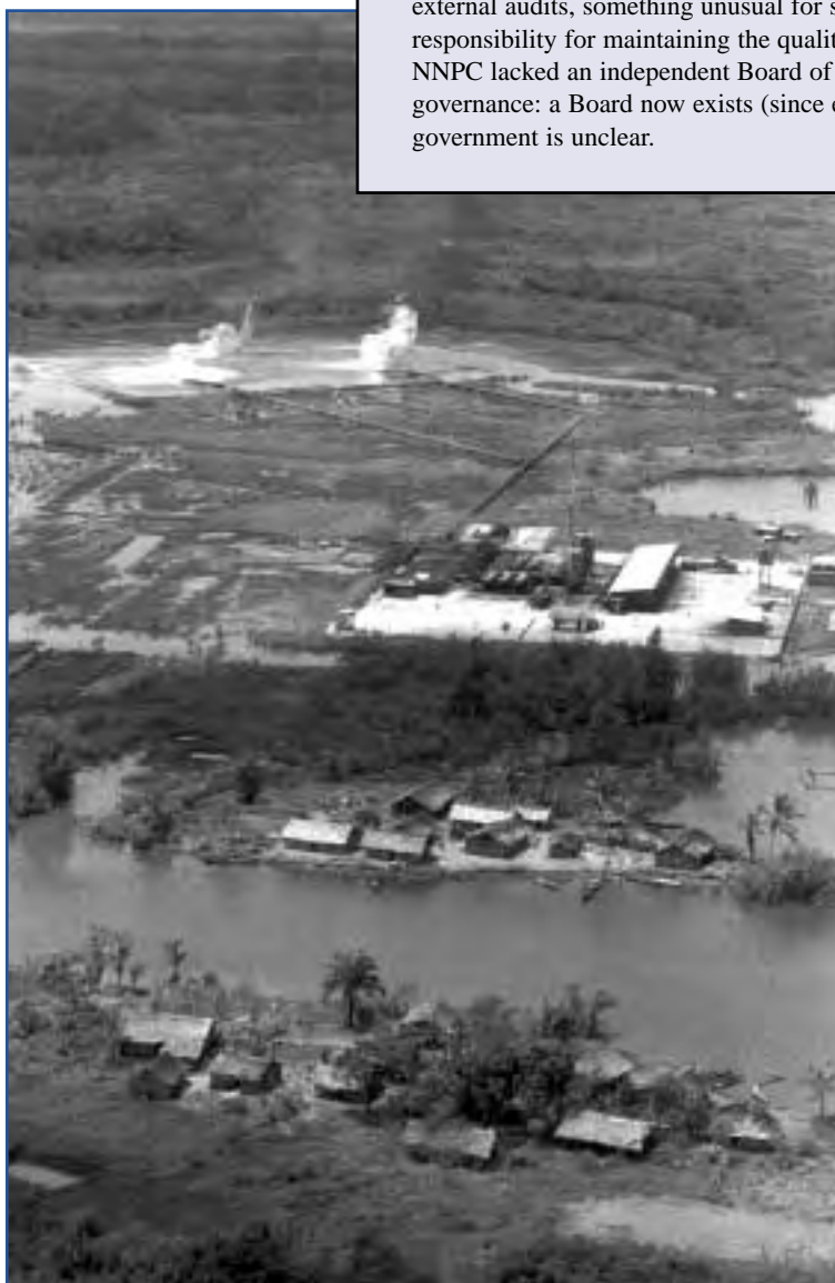
A Shell oil installation abuts villages in the Niger Delta, southeastern Nigeria. There is deep dissatisfaction in the Delta that Nigeria's massive oil wealth has not improved the lives of the local population. Occupation of facilities, political instability and theft of oil has cut production by up to one third in the last two years. (Photo: Africaphotos.com)
